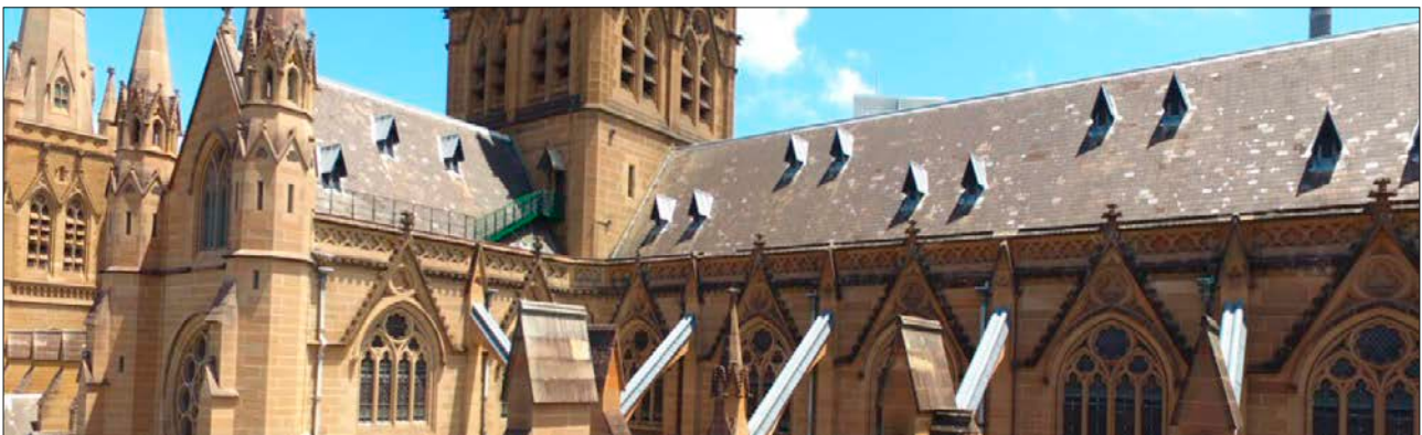
North East Roof of St Mary's Cathedral prior to restoration
