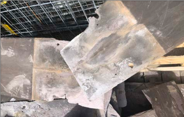
Damaged tiles from the 1800s removed
