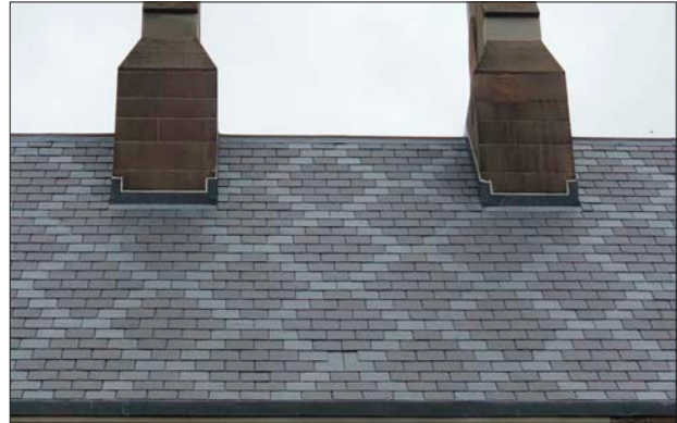
Retiled roof showing diamond pattern
