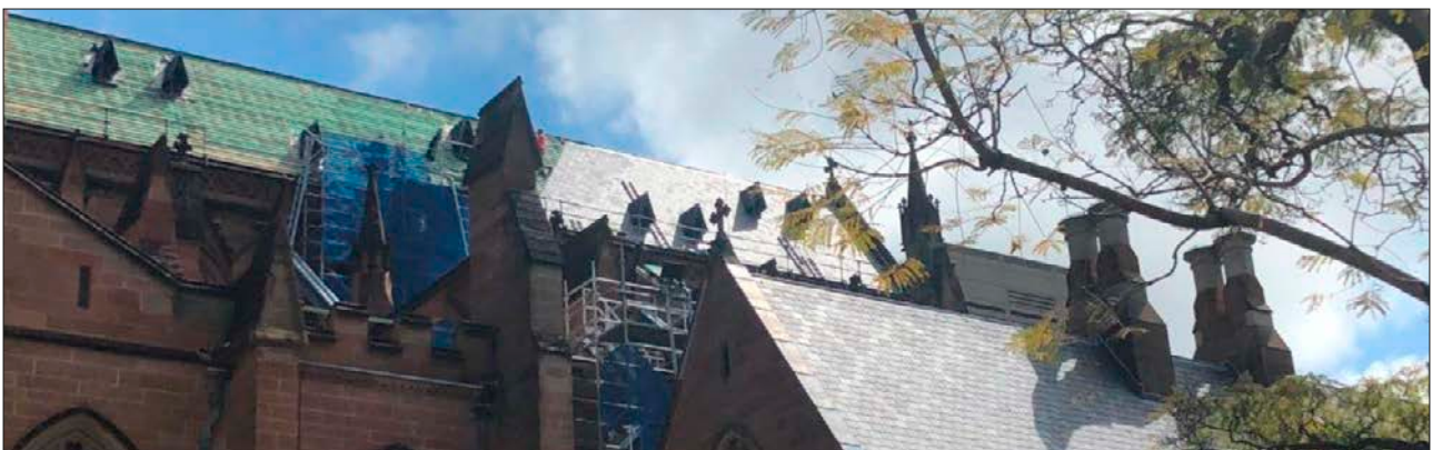
North East Roof of St Mary's Cathedral during restoration
